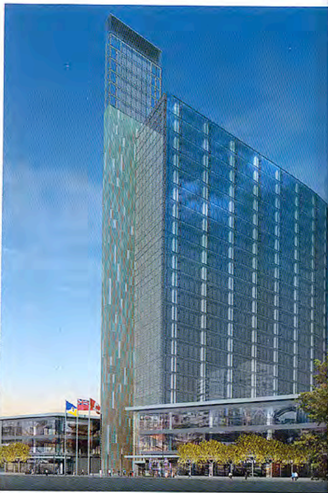
Manitoba Hydro Building: Above - North view, day. Page 13: Top - Atrium; Bottom - North view, night
